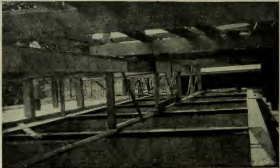
FIG. 3. CONCRETE TANKS FOR LOG BOILING.
